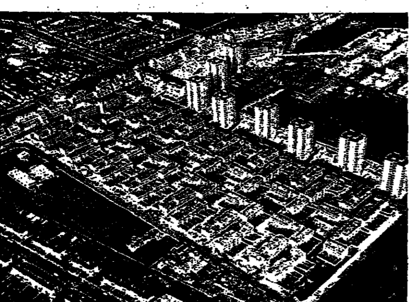
Thamesmead, planned as an 'infill' new town, in prosperous South-East England, is about 20 km. from London, on the south bank of the Thames. Begun in 1965 at an estimated cost of over £30m, the town is expected to be finished by 1980. It will accommodate 60,000 persons. (Camera Press)
